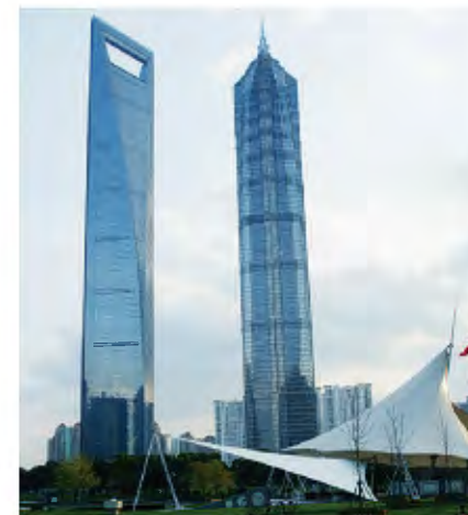
上海金茂大厦 Jin Mao Tower
